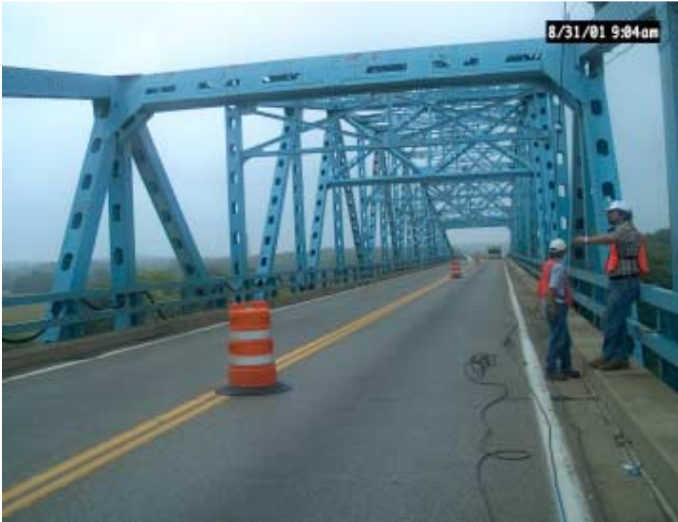
Figure 4. US 62 over the Cumberland River in Livingston County prior to painting.
